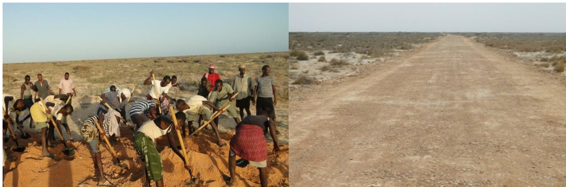
Hafun: Building a feeder road using labor intensive approach
